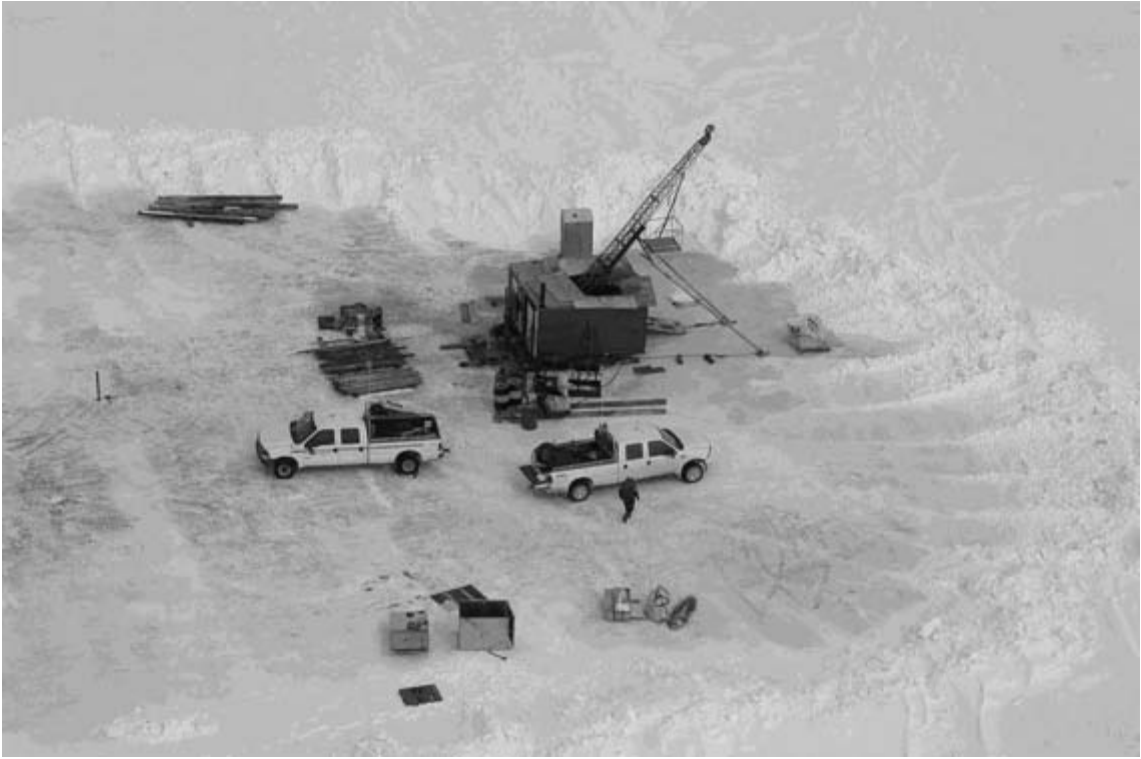
FIG. 17.18 Winter drilling. (Courtesy Diavik Diamond Mines Inc.)
